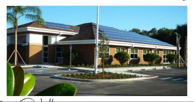
This energy-producing facility produces "net-zero" energy use, selling back energy to the utility company. Features include a rooftop solar panel system, porous paving for rain water absorption and daylight harvesting light sensors that direct outdoor light to the interior.
