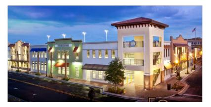
Led the design of a 260 space, downtown parking garage for the City of Winter Haven, Florida. The three-level, naturally ventilated commercial building is constructed of pre-cast concrete and uses LED lighting. The style of the surrounding downtown retail structures is reflected in the design of the street-facing walls.
