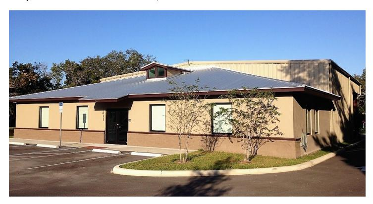
**3. Project Description:** 2,500 s.f. pre-engineered steel building warehouse with a 2,000 s.f. masonry office. Building is designed for storage of sales inventory of sports apparel for NFL, NBA, MLB and others, featuring climate-controlled humidity. The office portion serves personnel management and conference room activity.
